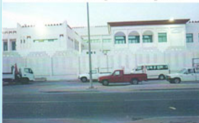
Hamed Bin Harbail Independent Secondary school at Najama Client : INSHA Contracting & Trading W.L.L.
