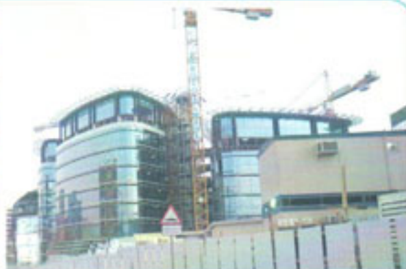
Business Park & Hotel Facility at Najama Client : REDCO Construction – Almana
